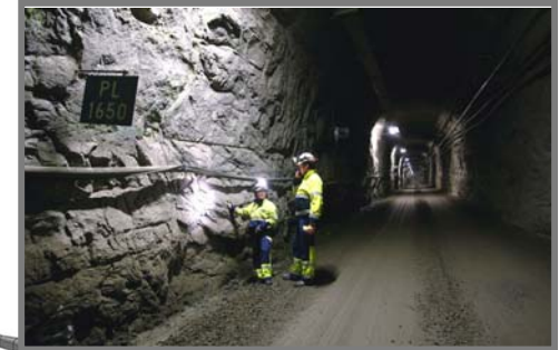
Access tunnel, 5 km
