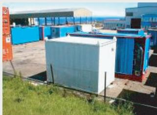
A60 Zone II offshore cabins with double thickness fire-proof steel wall,
