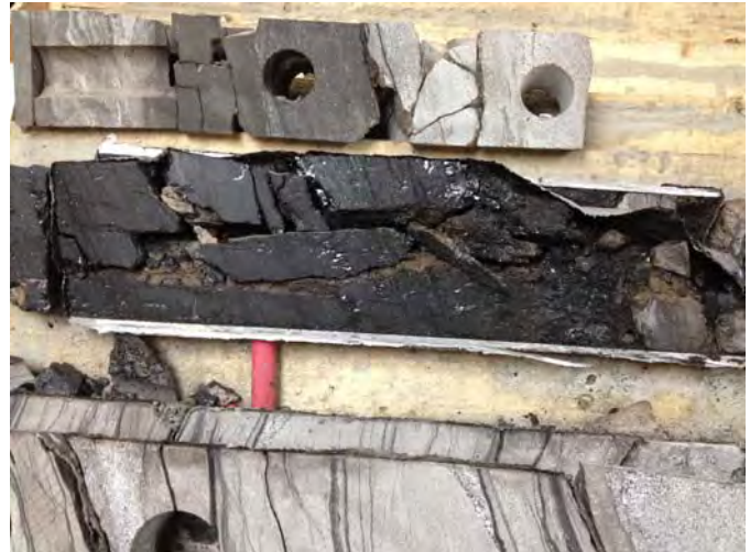
Even highly deteriorated material can be assessed
